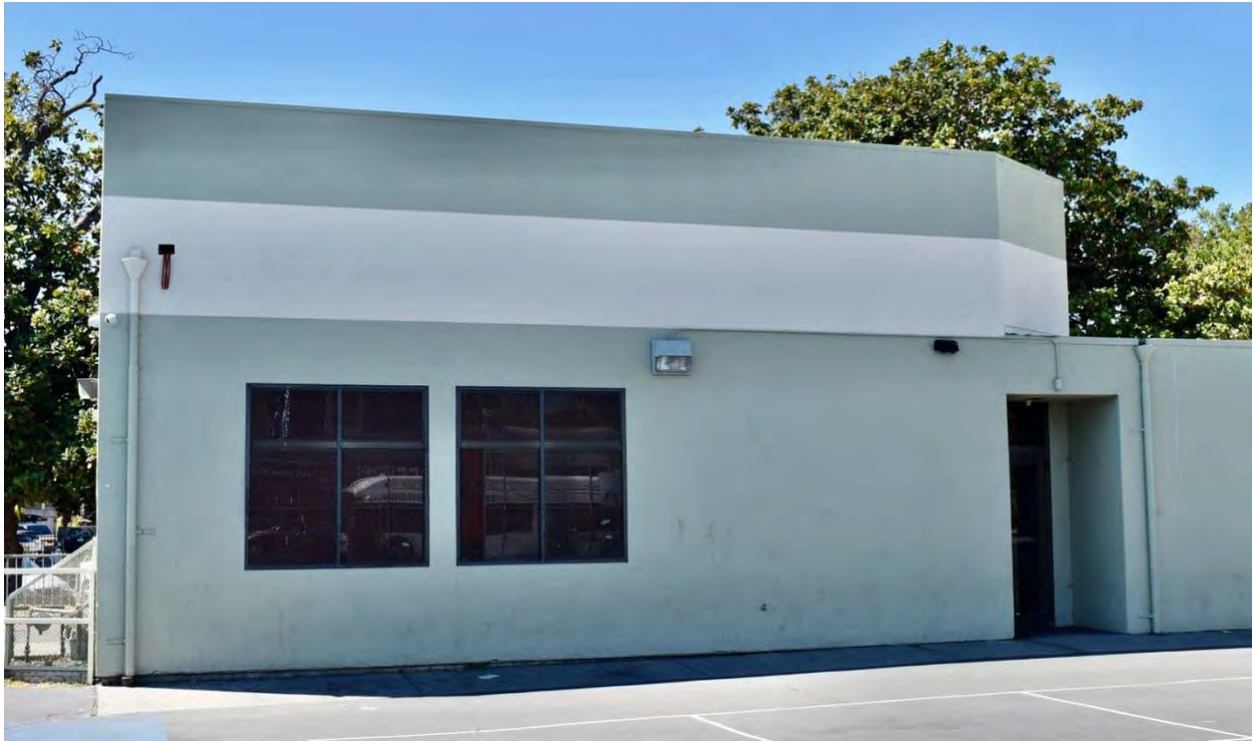
East wing, north façade
