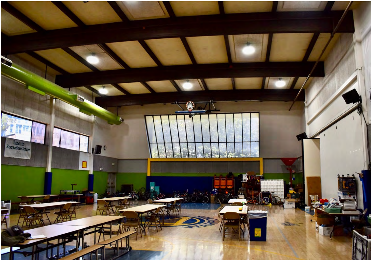
Figure 20: Multi-purpose room in west wing looking north
