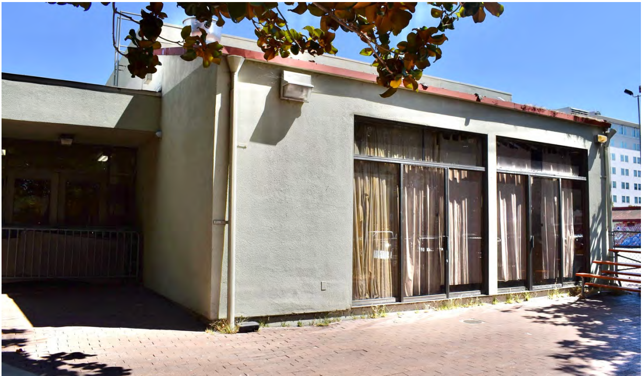
Figure 13: East wing, south façade
