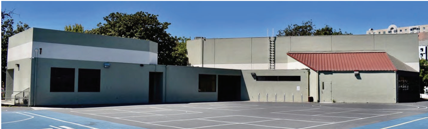
Photo 1: Existing Lincoln Square Recreation Center, North and Northeast Façades
