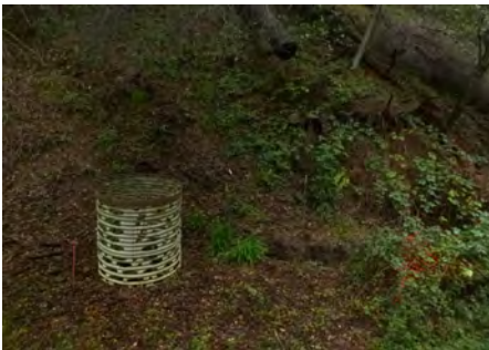
Beaconsfield Canyon Storm Drain Inlet Replacement
