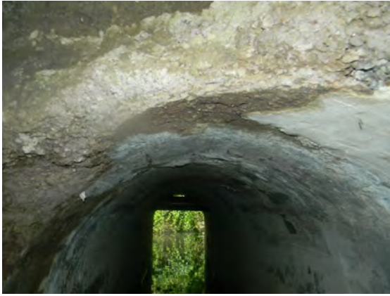
Richmond Blvd. Stormwater Culvert Repair
