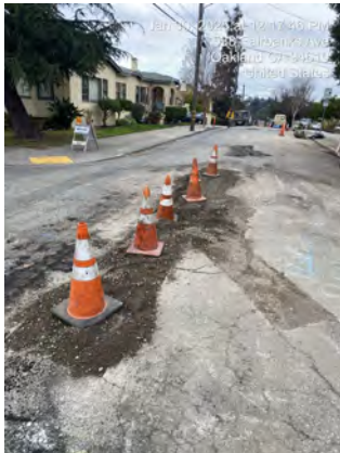
Sanitary Sewer Rehabilitation - Sub-Basin 85-211
