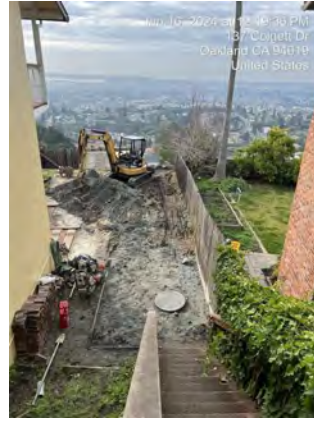
Sanitary Sewer Rehabilitation - Sub-Basin 85-102
