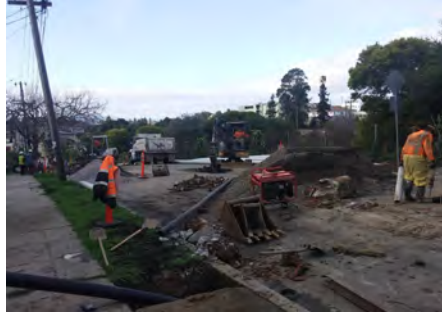
Hotspot Sewer Repair
