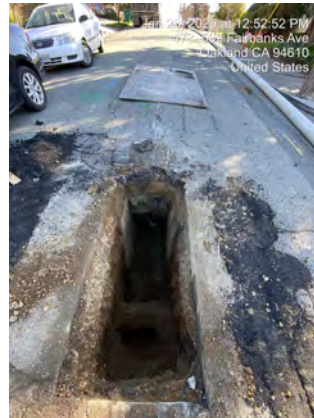
Sanitary Sewer Rehabilitation - Sub-Basin 85-231
