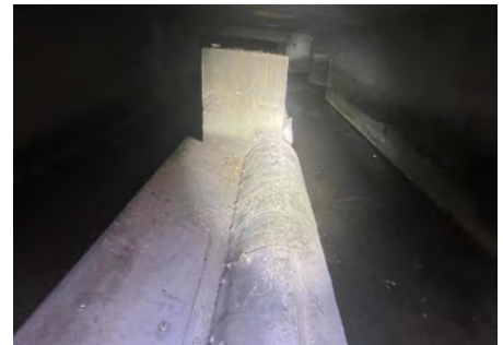
Broken Weirs Replacement - 73rd & International Large Capture Trash Device
