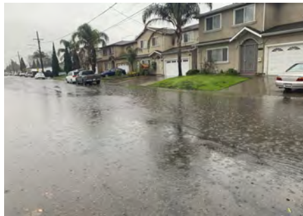
Bernhardt Drive Storm Drain Improvement
