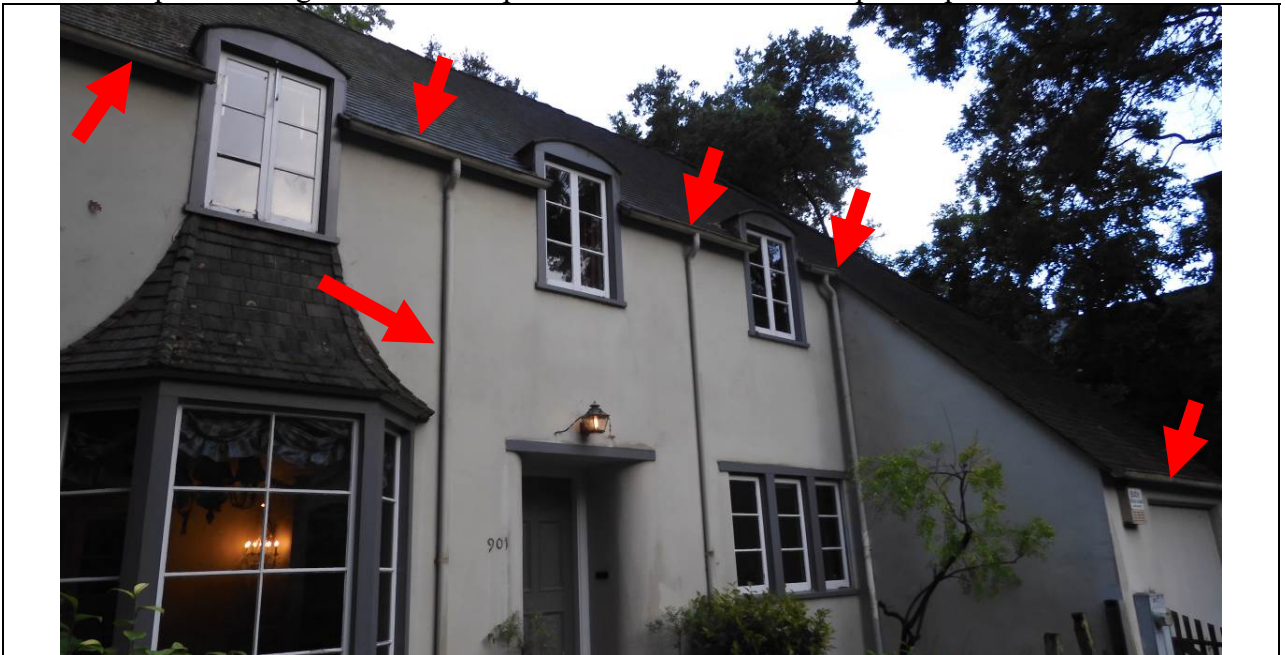
Work Item #7 - Photo 1 Historical gutter and downspouts to be repaired and/or replaced.
