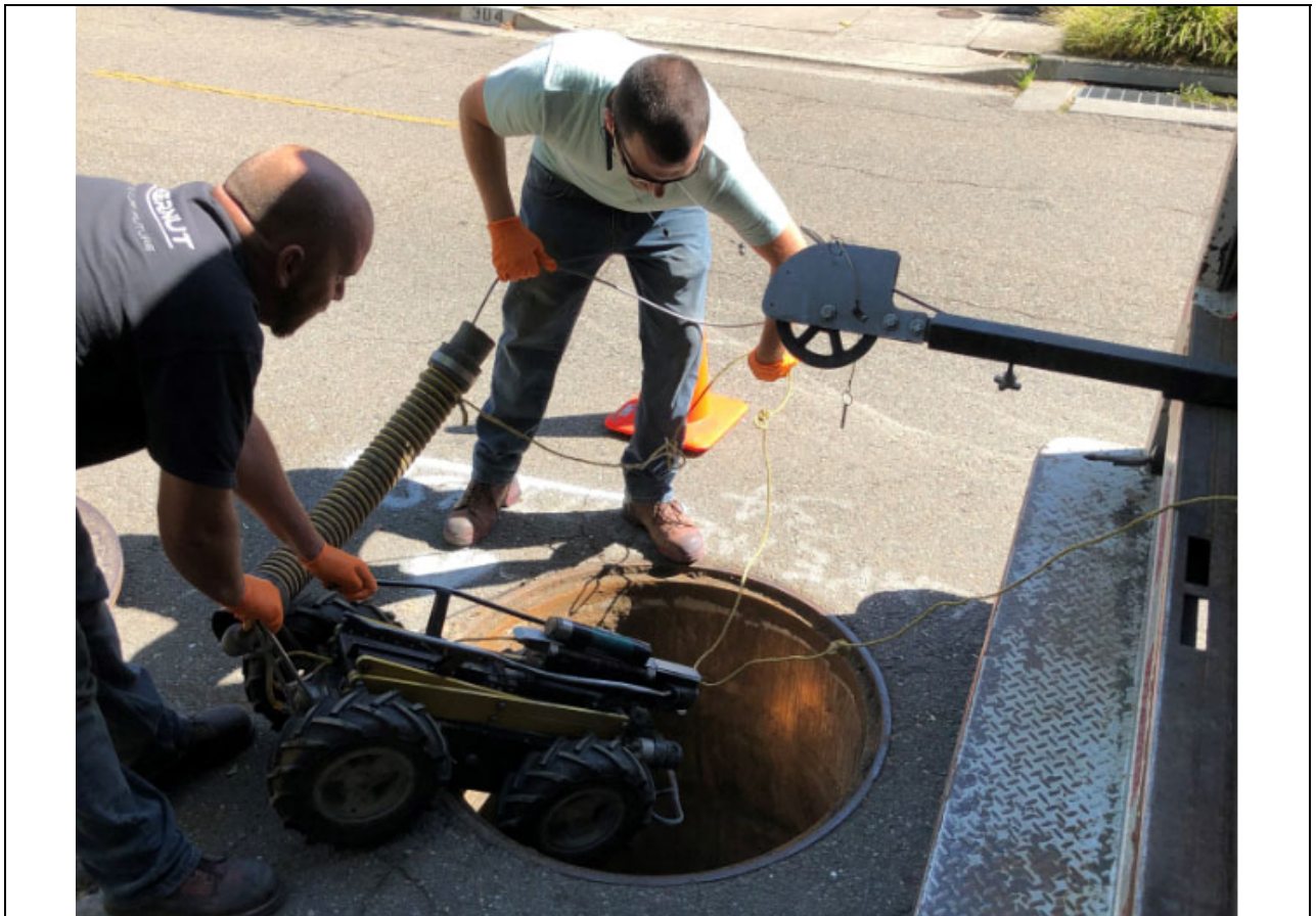
Work Item #1 - Photo 2 Robot with camera entry into Trestle Glen Road culvert access port directly in front of 901 Trestle Glen Road (2019).
