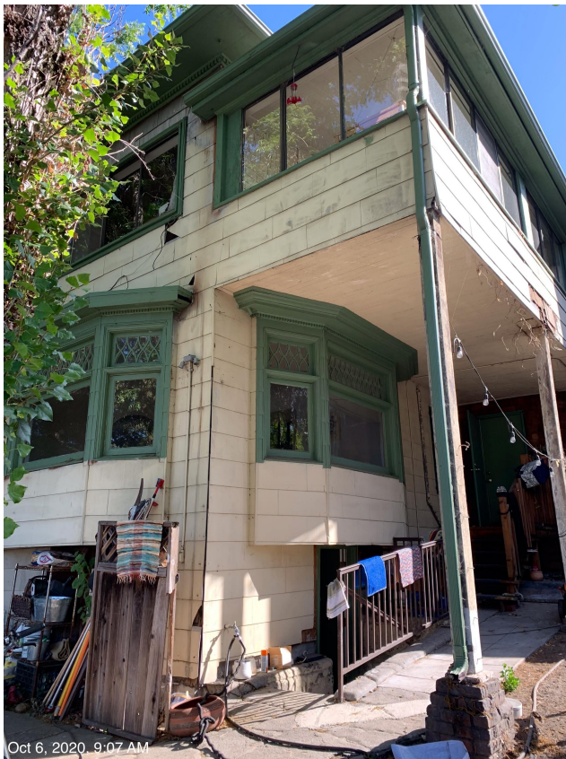
back porch which will be held up by a hardy frame, notice the brick foundation under the wood columns
