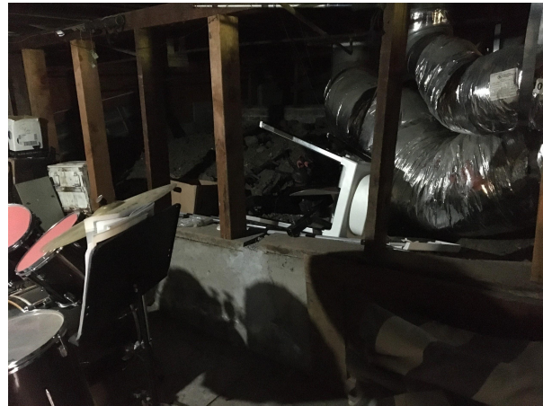
shear panels to be added to cripple walls, current support beams are leaning
