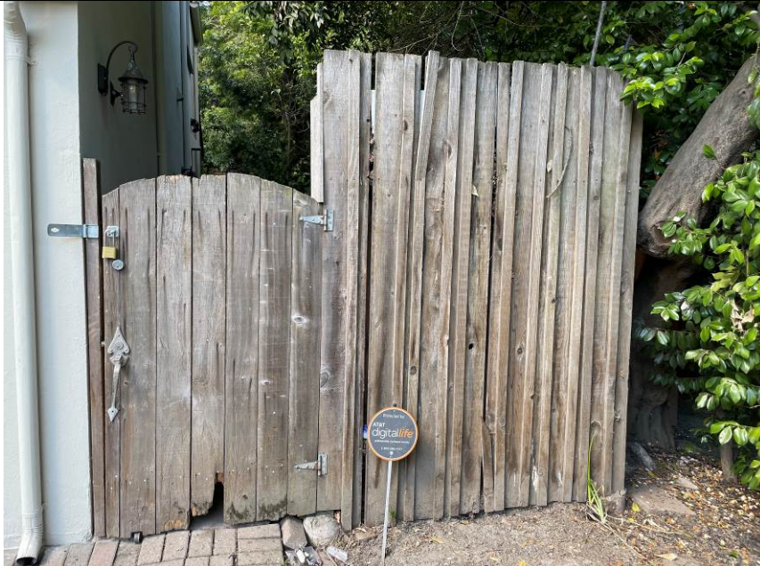
Work Item #3 - Photo 2 Right front garden fence front elevation. Fence has wood rot and missing panels.
