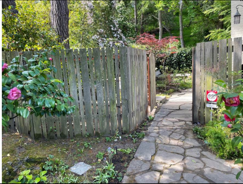
Work Item #3 - Photo 1 Left front garden fence between the house and Warren Hook Park. Current fence has wood rot and missing panels.
