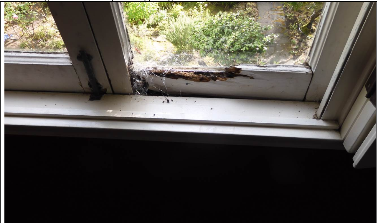
Work Item #2 - Photo 1 Second Floor Window with dry rot and slipping window panes.
