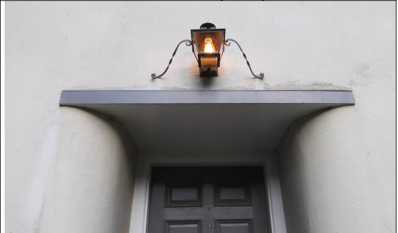
Work Item #2 - Photo 6 Remove repair and rewire original light feature. Exposed wire insulation present. Patch and paint exterior wood and stucco.
