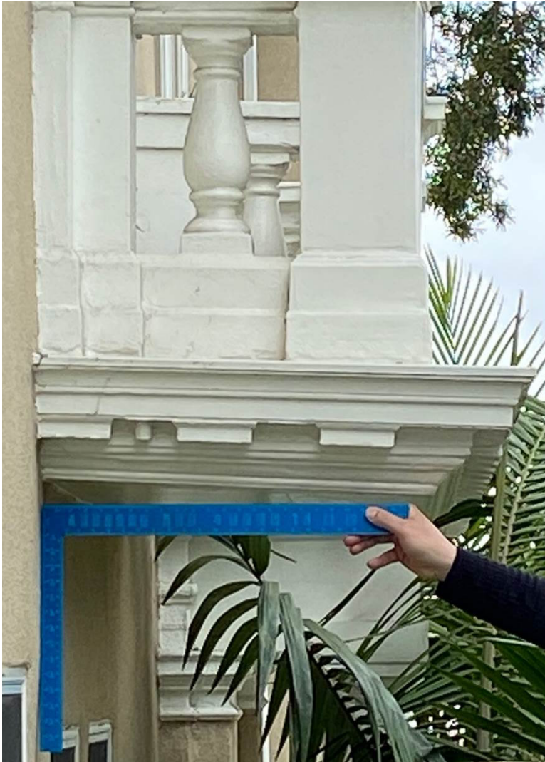
Work Program Item #3 Figures A, B and C: Restoration of Cantilevered Balconette
