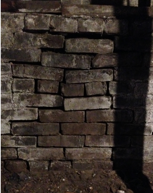
Fissures in the brick foundation
