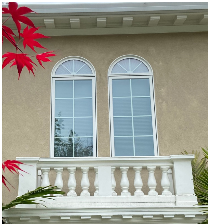
Work Program Item #2 Figure B: Two full-height narrow casement windows with overlying fanlights
