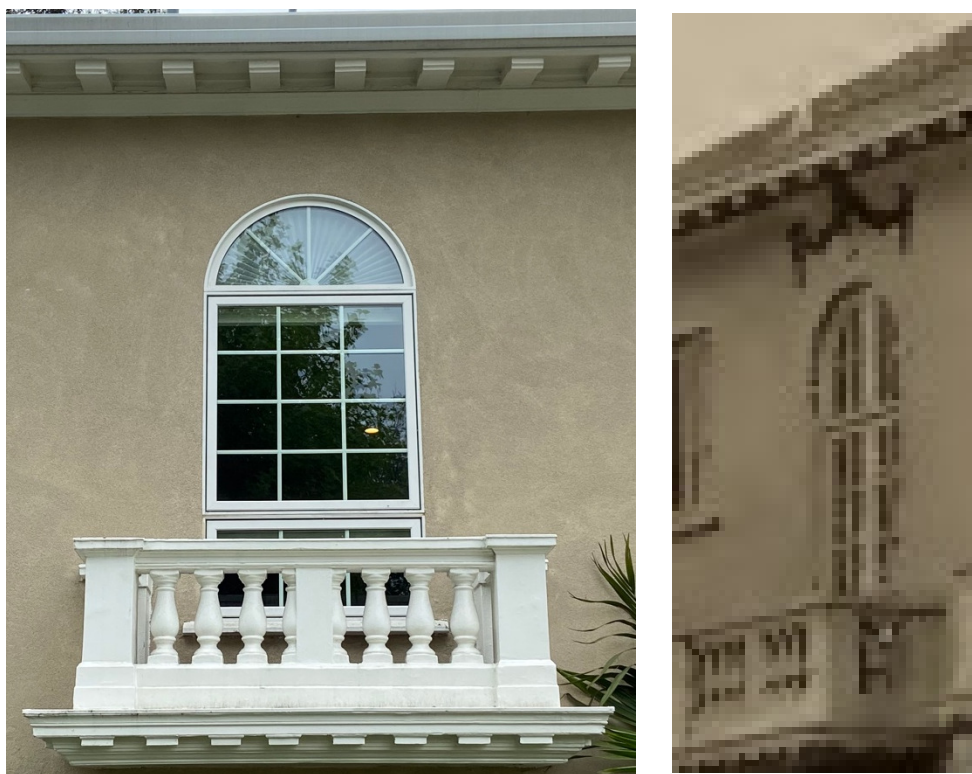
Work Program Item #2 Figures C and D: Eastern-most (left) cantilevered balconette partially obscuring large fanlight, square fixed window, and rectangular fixed window. French windows with an incorporated semicircular arch were featured in the original design (right)
