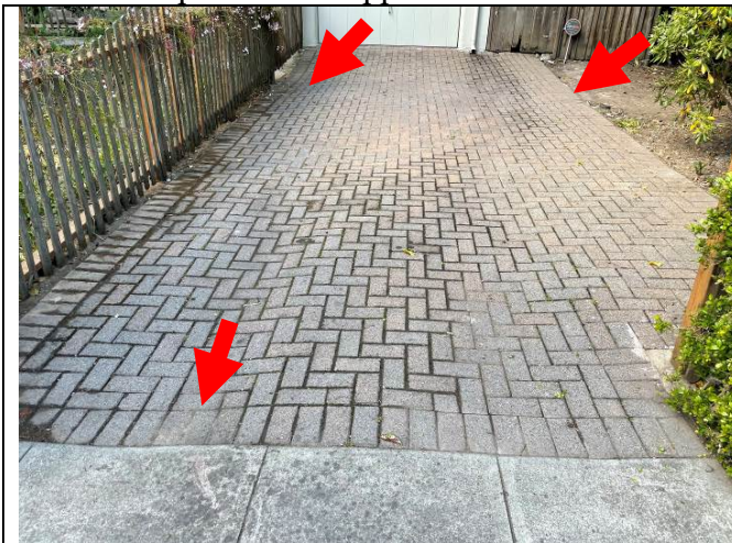
Work Item #9 - Photo 1& 2 1990's era concrete brick driveway to be repaired. High spots and valleys are present. Sewer line underneath to be replaced. (If this was concrete it would be severely cracked but the brick helps conceal the soft sediment deformation. Exposed utility box.
