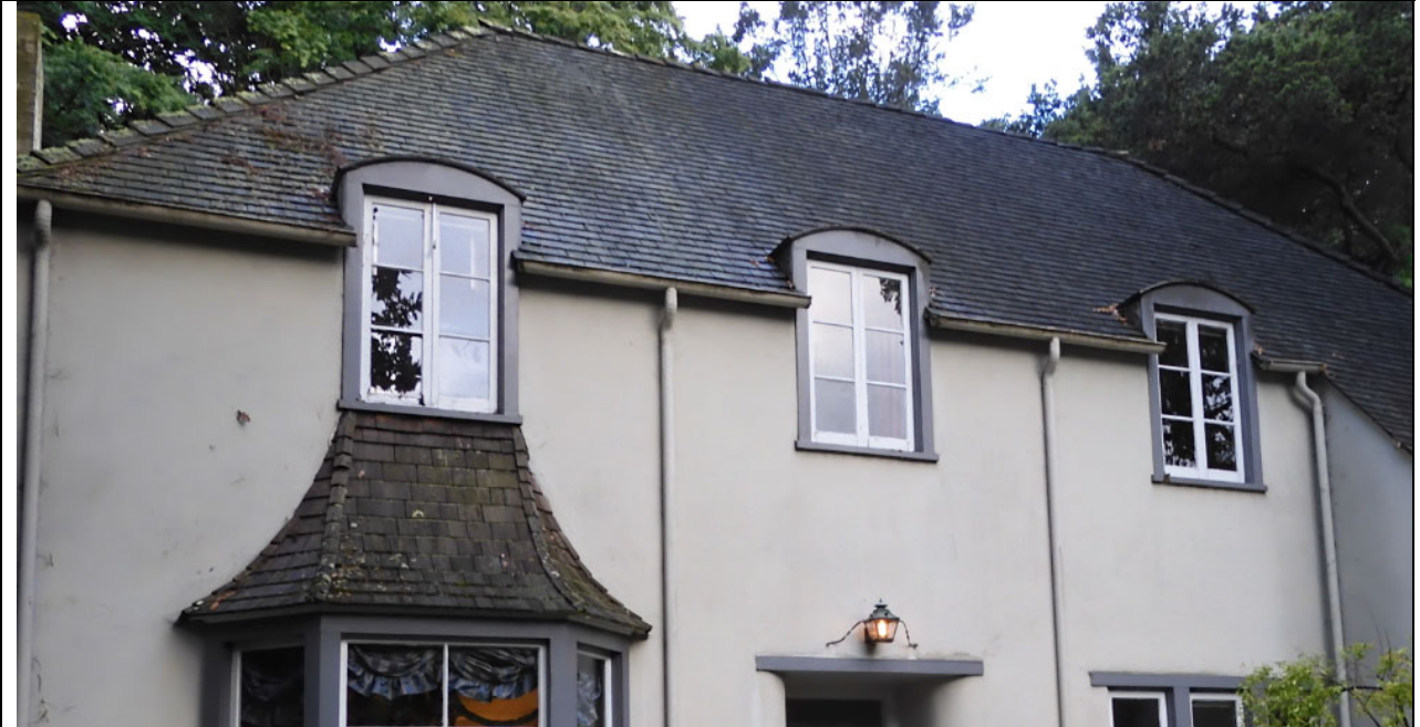
Work Item #4 - Photo 1 Replace wood shingle roof with new fire-retardant rated wood shingle roof on upper & lower portions. Wood roof dated early 1990s.
