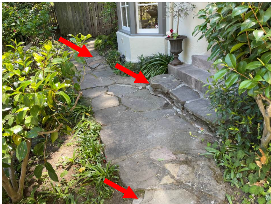
Work Item #4 - Photo 3 Red arrows show missing and or significant separation based on ground settling.
