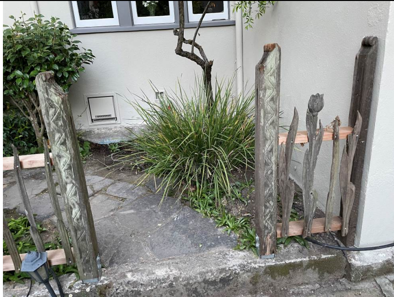
Work Item #2 - Photo 3 Example of rose garden fence and posts carved and mounted to the house. Several fence items are damage or missing.
