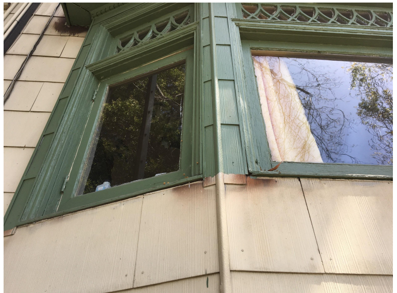
notice the detail work, small asbestos shingles between the windows, original window trim surviving in part
