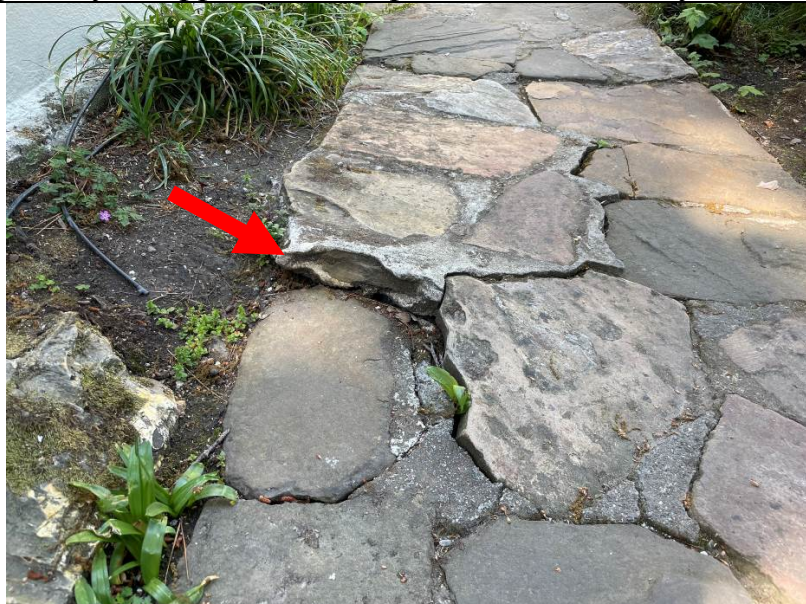
Work Item #4 - Photo 2 Red arrow depicts significant separation based on ground settling.
