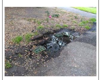
Leaking irrigation and erosion on the East side of the Park near Broadway
