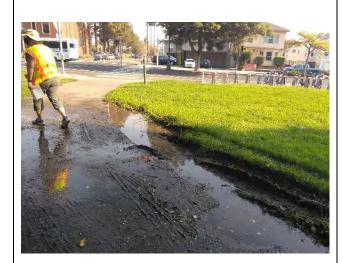
Leaking irrigation and erosion in the North Central part of the park facing MacArthur Blvd
