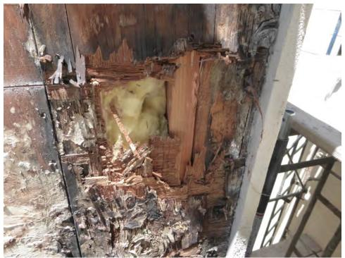
More of the same extending down the building corner causing dry rot and severely compromising the structural sheer.
