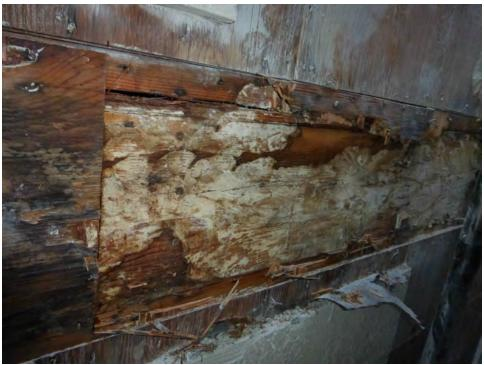
Moisture damage and fungal growth traveling along rim board behind plywood sheer.
