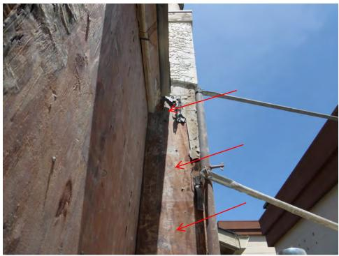
Evidence of water intrusion at chimney chase directly below roof/chimney chase wall juncture.
