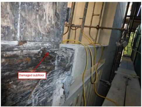
More of the same. Noted dry rot damage at subfloor possibly extending into the unit.
