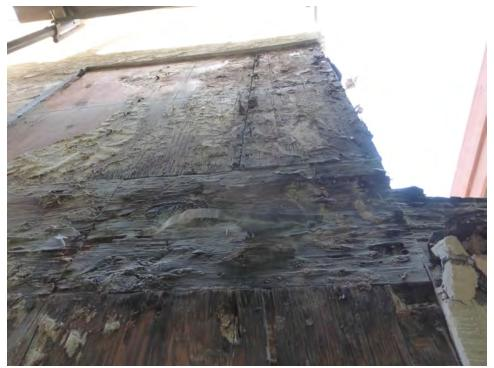
Severe dry rot noted at the upper lateral support beam as a result of missing roof related and beam/wall juncture flashings.
