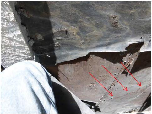
Minor evidence of water staining at sheer plywood midway between roof and upper lateral beam.
