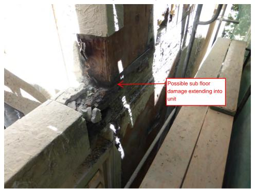
More of the same extending to exposed lateral beam. Noted dry rot to sub-floor and possibly continuing into the unit.
