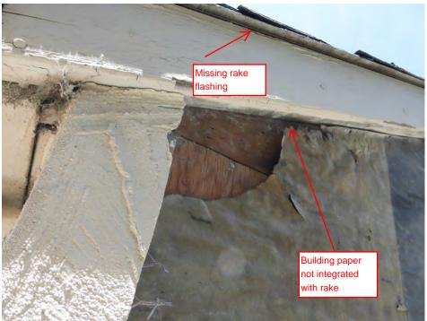
Evidence of water intrusion was noted as a result of missing roof rake nosing and non-integrated building paper similar to conditions found at the east corner.
