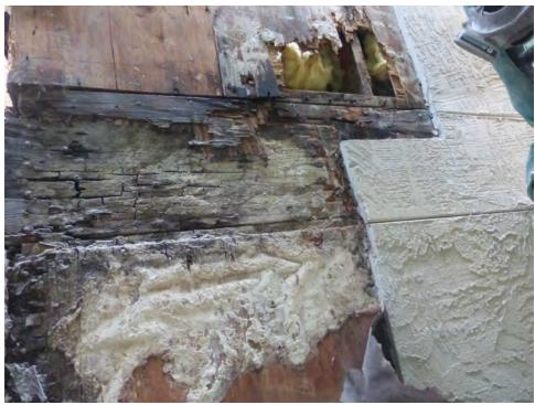
Severe structural damage appears to be related to improper stucco control joint installation. Similar condition present at south east corner of the building.
