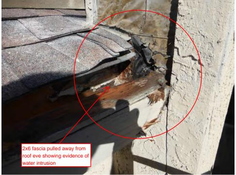
Missing roof edge flashing, gutter and diverter allowing water intrusion at confined rake of chimney chase.
