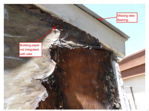
During the investigative removal process, evidence of water intrusion was noted as a result of missing roof rake nosing and non-integrated building paper.
