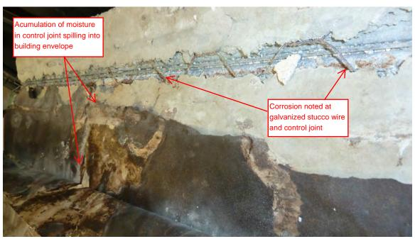
Example of stucco control joint installed directly over stucco wire creating a path for moisture, breaking down building paper and allowing infiltration into the building envelope.
