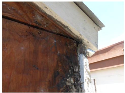
Lack of roof/wall integrated waterproofing allowing moisture infiltration behind building paper.
