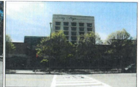
2: Rear (south facade) neighbor, Laney College, from the southwest corner of the building.
