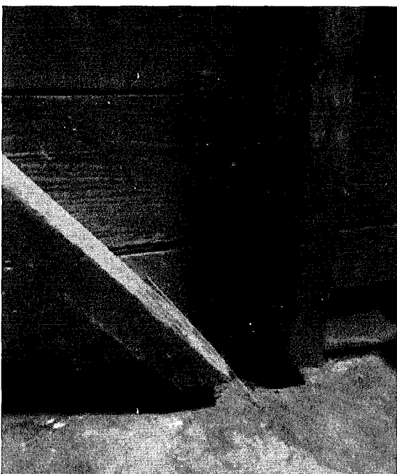
Garage separating from foundation
