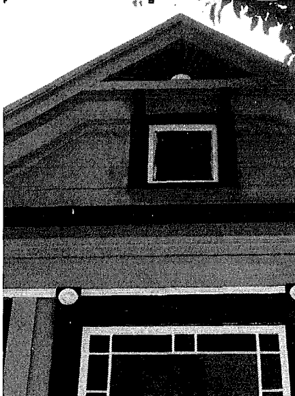
Asbestos siding beneath the sunburst, probably covering shingles; damage to wood siding
