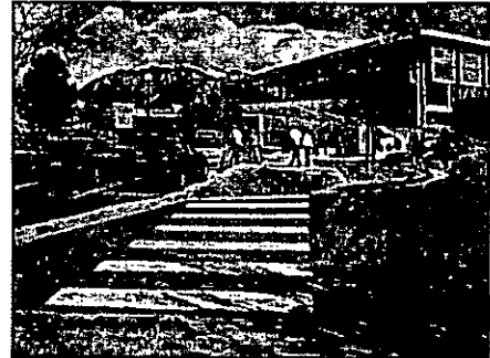
Example of pedestrian pathway (crosswalk and sidewalk) to main building entry
