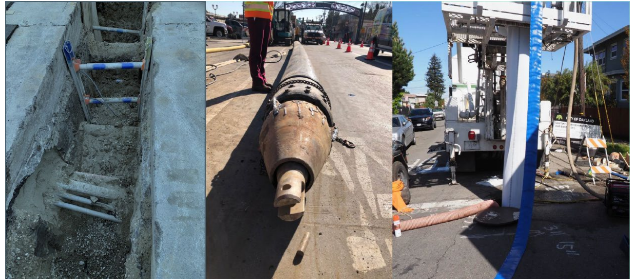
Open Trench | Pipe-Expanding | Cured-In-Place
