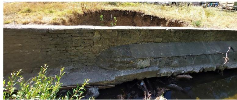
December 2021 storm undermined Sausal Creek retaining wall and eroded hole in Dimond Park lawn. Large hole repaired in fall 2022, repaid damaged by 12/31/22 storm.
