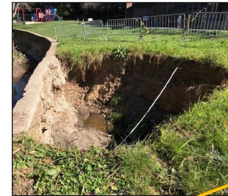
Capacity of downstream culvert will continue to cause flooding of Dimond Park in large storms which are becoming more frequent due to climate change
