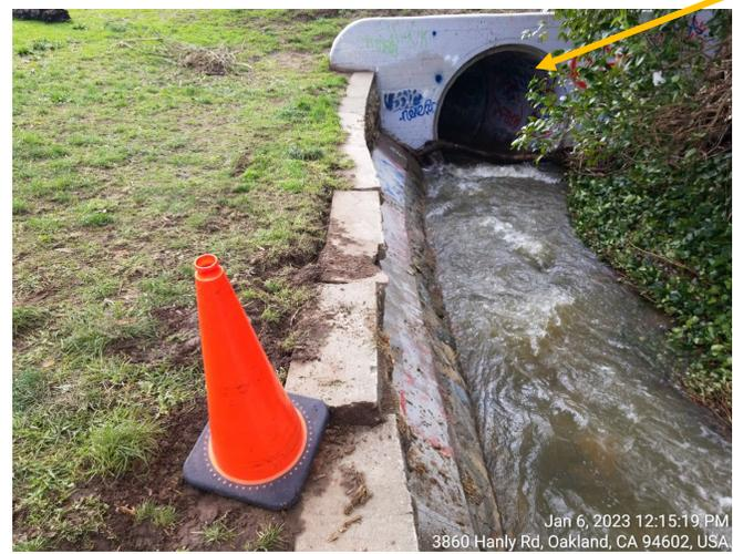
12/31/22 flooding further damaged retaining wall.
