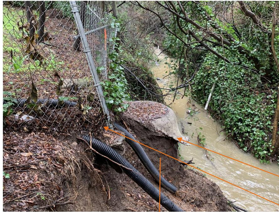
Exposed sewer manhole due to creek bank erosion. Fence at 6251 Hillmont Drive boundary may be encroaching into City ROW
