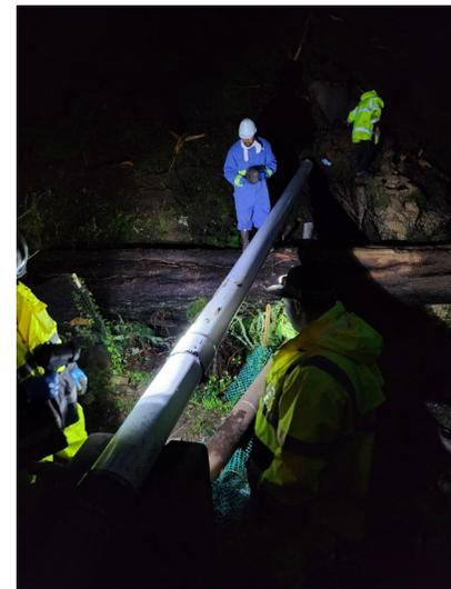
Broken sewer line from fallen tree caused by landslide in severe winter storm.
