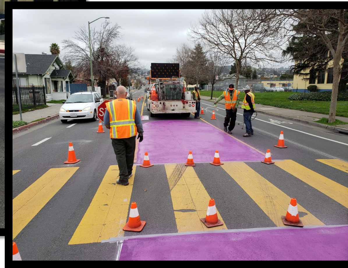
98th and Cherry Safety Improvement Project (near term improvement later installed with concrete)
