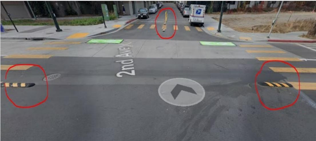
Hardened centerline treatment extending into the intersection
