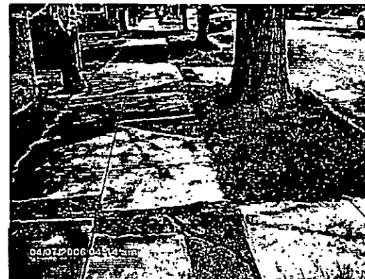
Tree Damage to Sidewalk
