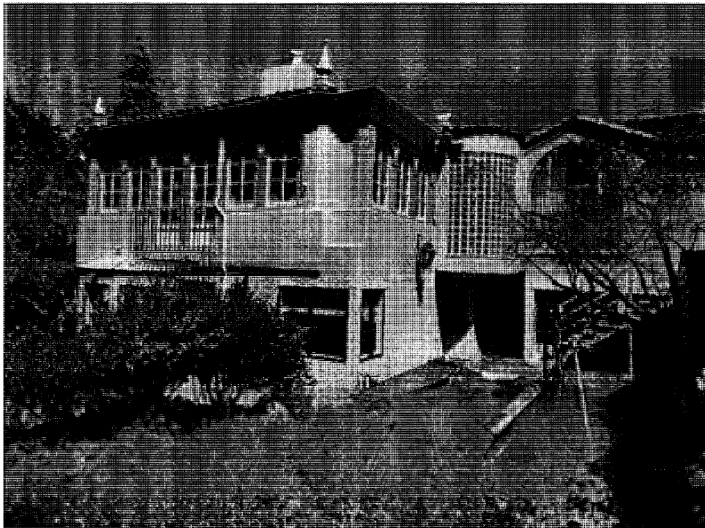
Figure 22. Overview of south façade, view north (SWCA, 2018).
