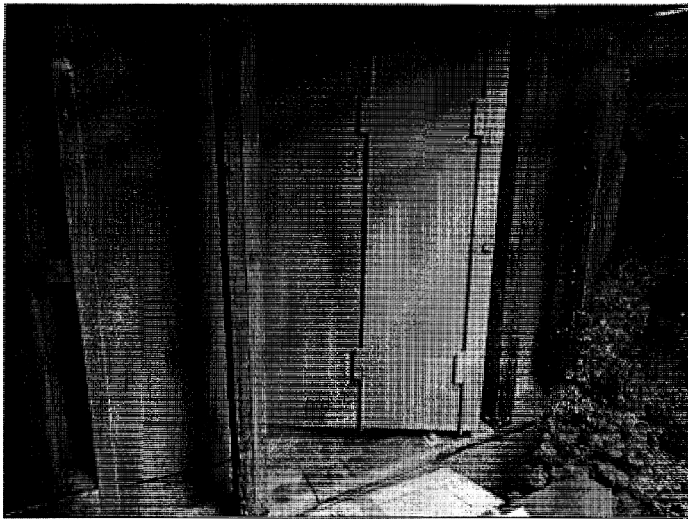
Figure 29. Steel cabinet in basement storage room, view east (SWCA, 2018).
