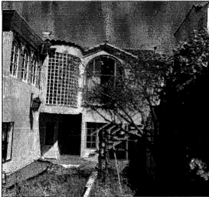
Figure 66. Detail of upper patio south of garage, view north (SWCA, 2018).
