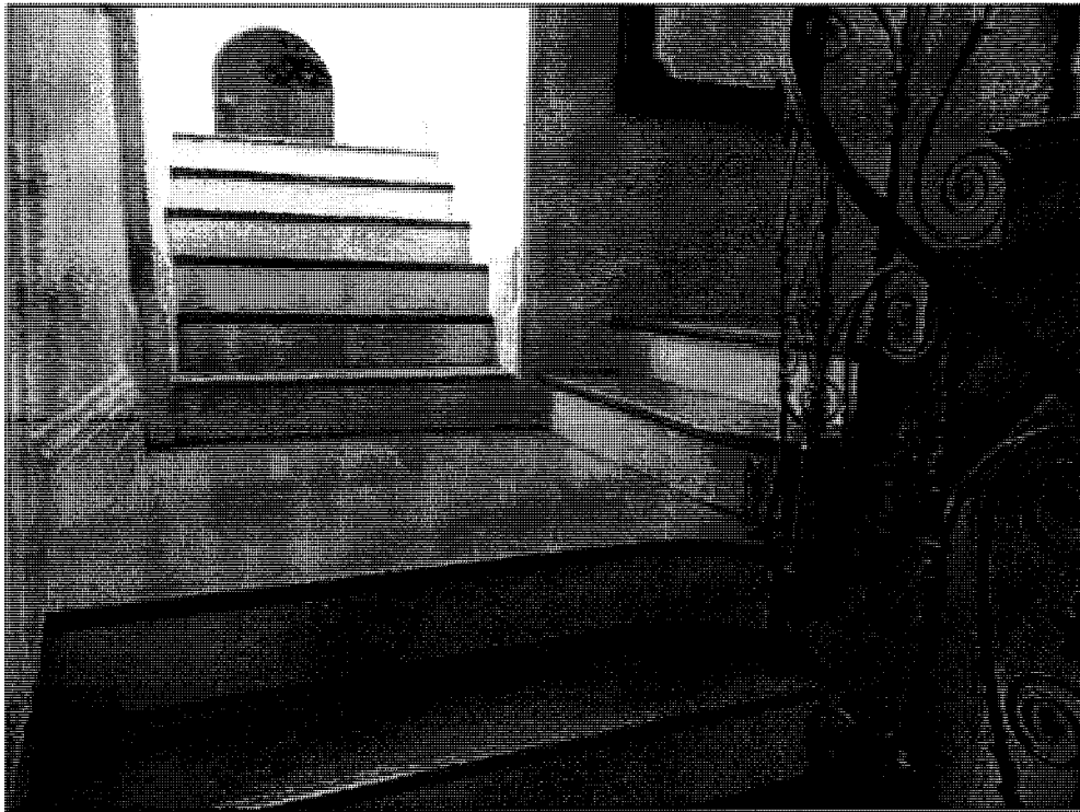
Figure 44. Second-floor landings, view east (SWCA, 2018).
