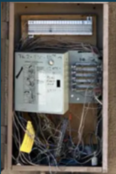
ISP-owned copper cable interconnects with CAT3 house cable
