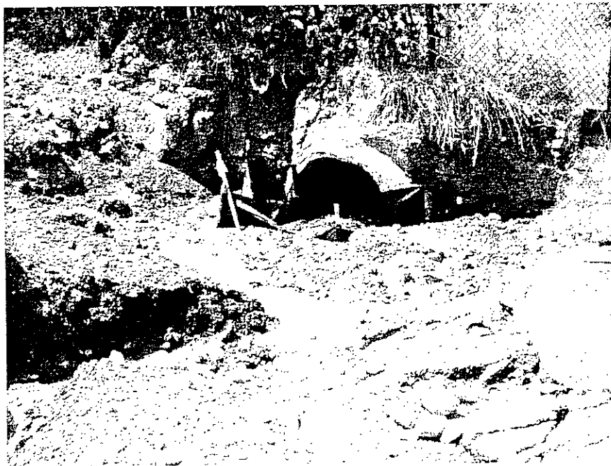
Same storm drain showing discharge during previous rain in July 2004.
