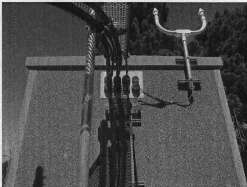
EBRCS Shelter at Seneca Reservoir
