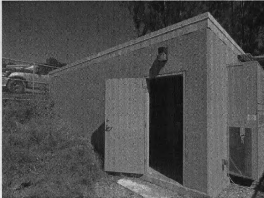
EBRCS shelter at Berkeley Labs
