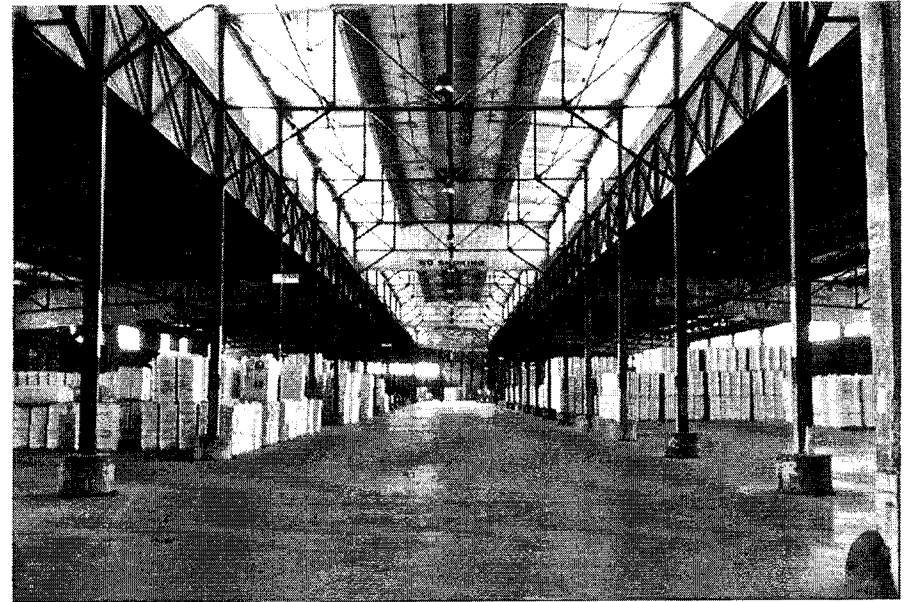
Metal trusses and columns offer reuse opportunities for artistic works and furnishings
