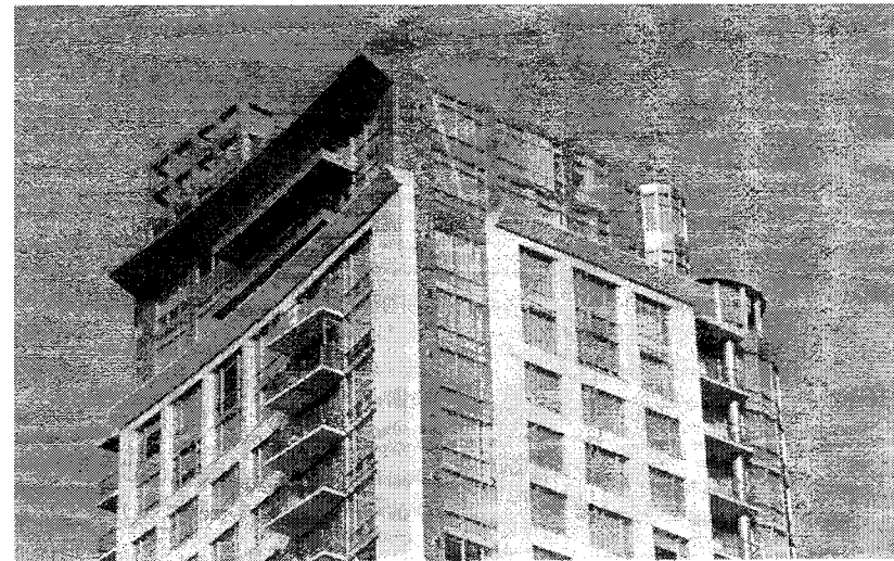
The topmost floors of towers should be architecturally differentiated through the use of setbacks, changes in material, building shape, etc.
