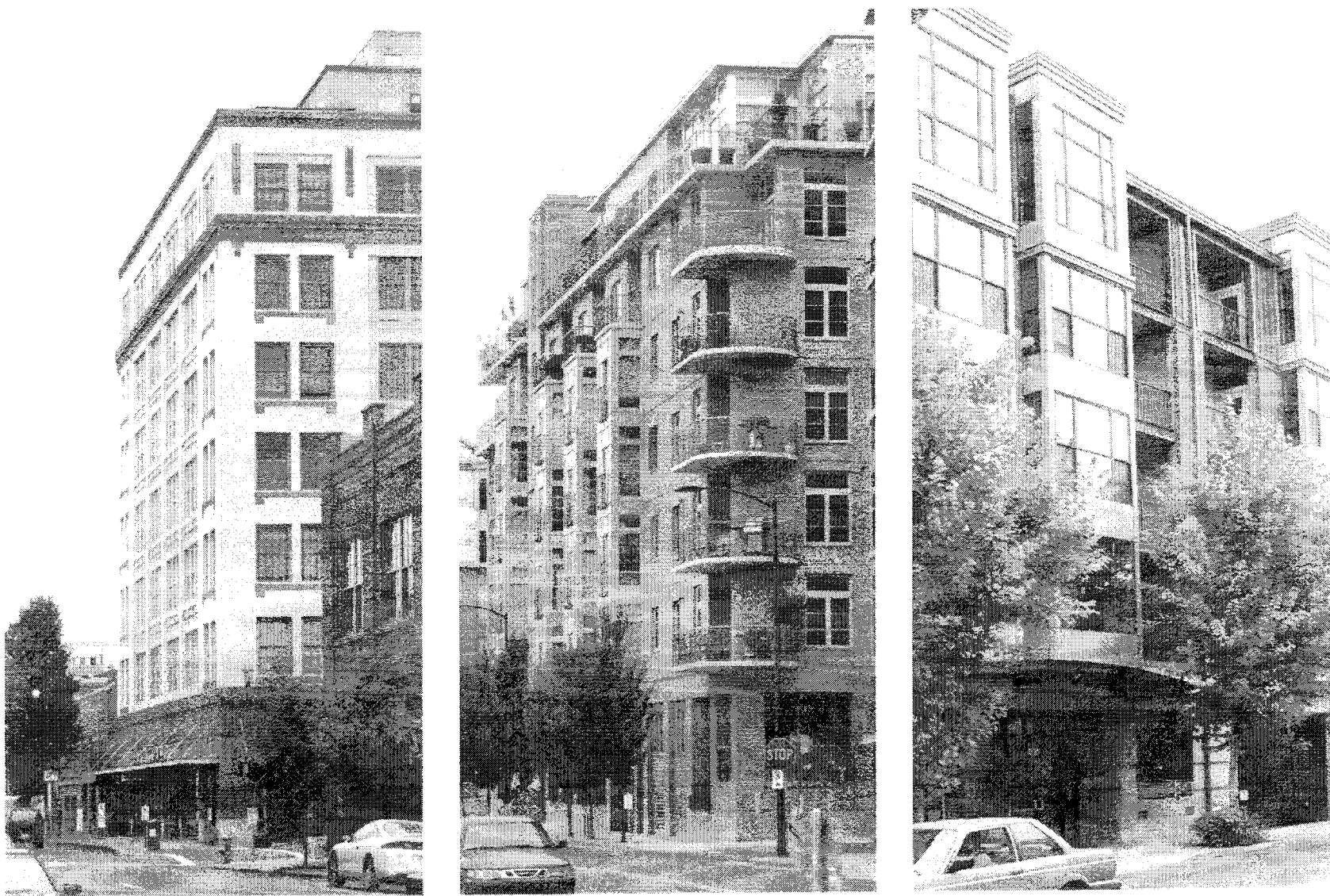
Buildings should introduce a differentiated architectural expression and/or a stepback of at least 5 feet above a height of 65 feet. Varied fenestration, balconies, bay windows, loggia etc., are encouraged to promote variation and articulation along streetfronts.
