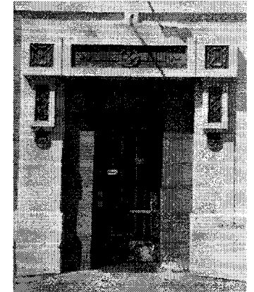
FRONT DOOR DETAIL
