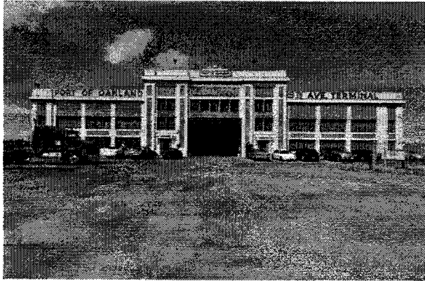
FRONT OF BUILDING
