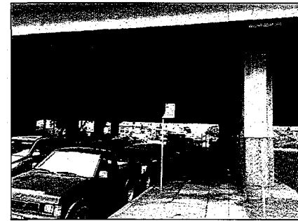
A VIEW NORTH-EAST TOWARD 6TH ST
