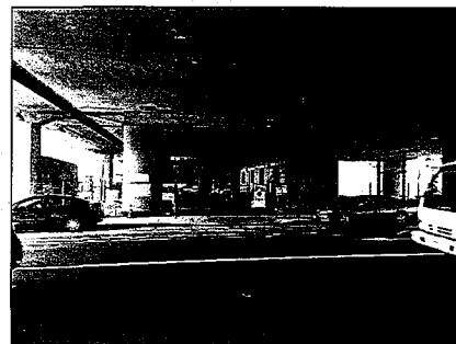
A VIEW ACROSS MADISON ST, UNDER I-880
