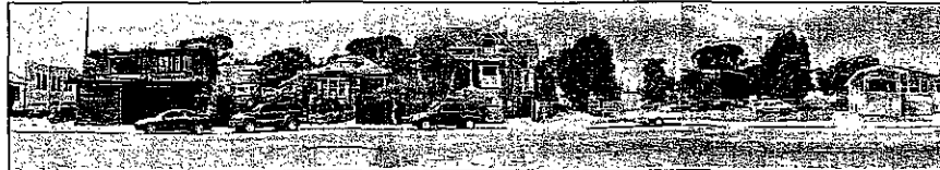
4801 SHATTUCK AVE PROJECT SITE
