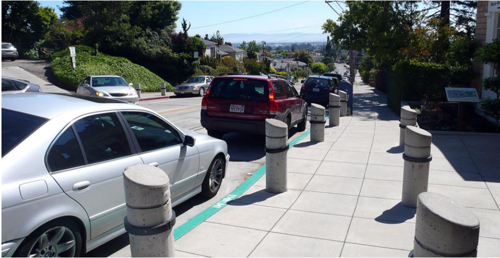
Figure 1-3 Campus Access – Photo Looking West on Lincoln Avenue (Sidewalk & Drop-off)
