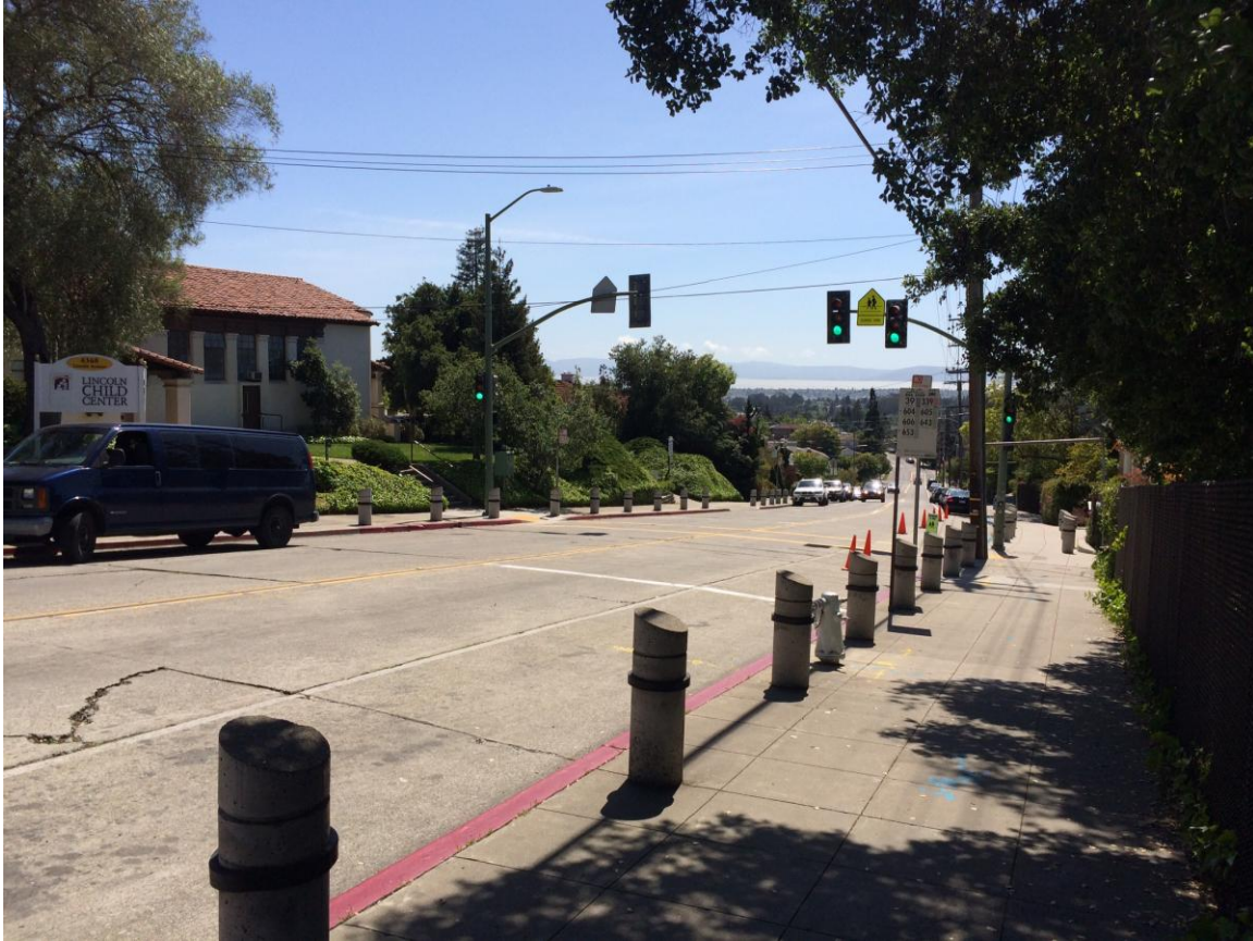
Figure 3-1 Existing Sidewalks –Photo Looking West on Lincoln Avenue
