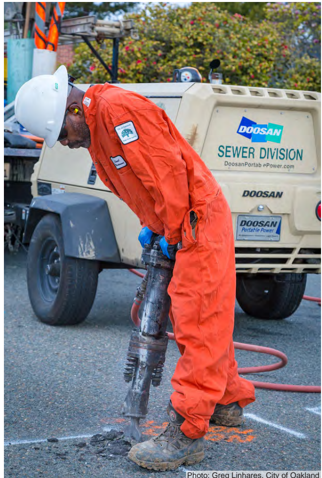
Photo: Greg Linhares, City of Oakland
