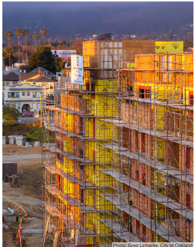
Photo: Greg Linhares, City of Oakland
