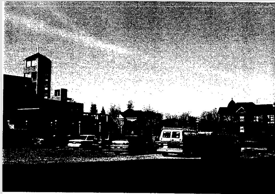
Figure 1-4 Existing Block T10 Site Conditions
