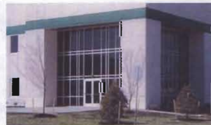
Example of window articulation
