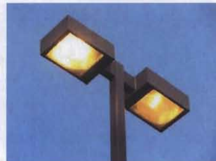
Example of light fixture with shielding
