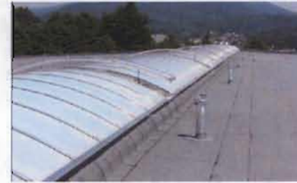
Example of skylights
