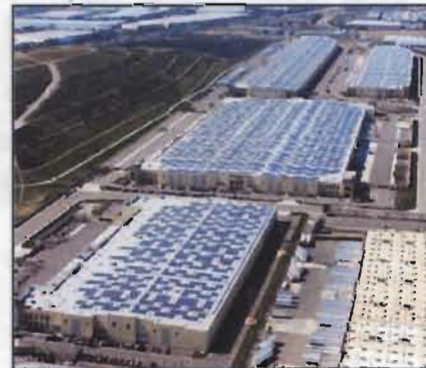
Example of rooftop solar panels
