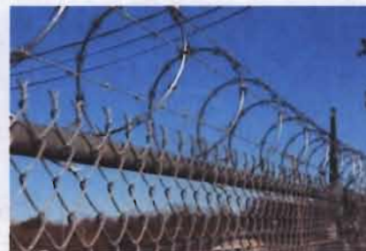
Barbed wire and razor wire are prohibited
