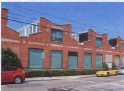
Example of historic building with articulated shape
