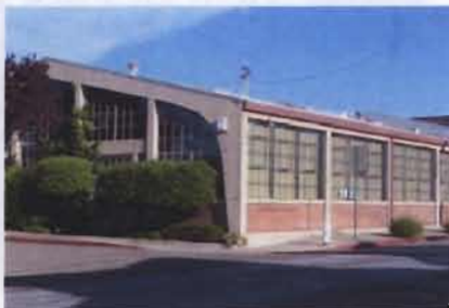
Example of industrial materials – masonry, concrete and glass
