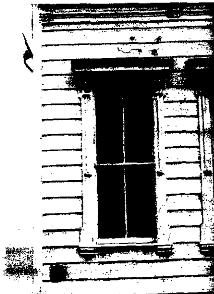
Photograph 17. Exterior window at 1970 San Pablo.
