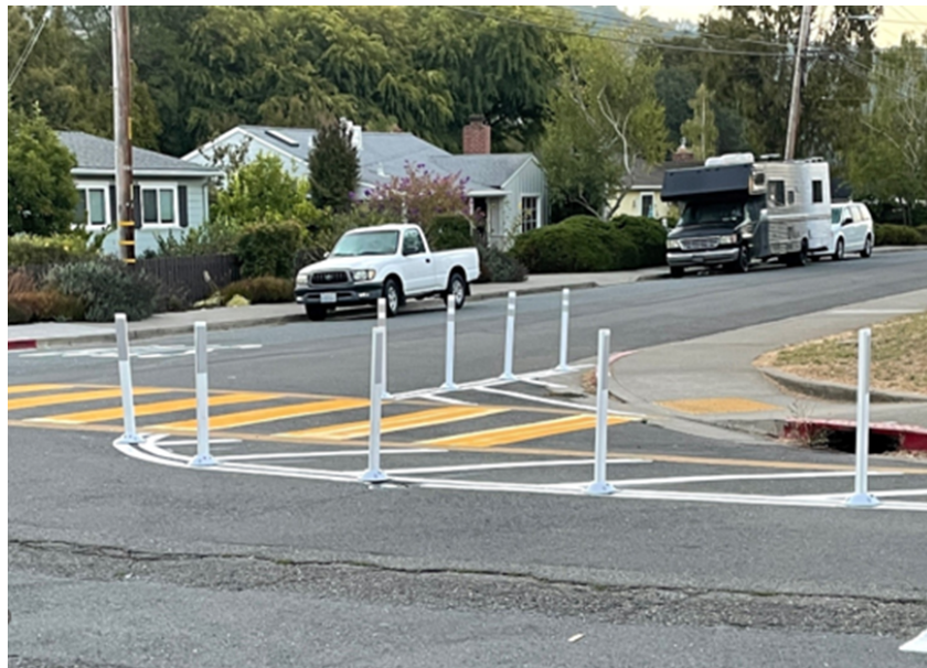
Figure 2 - Curb extension example, Redwood Heights Elem School, 39th Avenue and Reinhardt Drive
