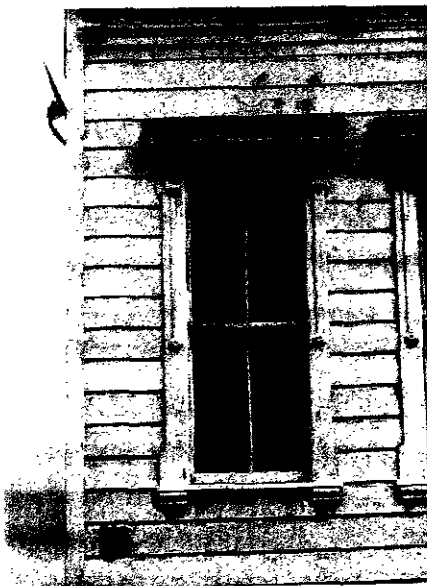
Photograph 17. Exterior window at 1970 San Pablo.
