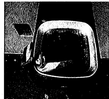
Poplar-leaves plugging drain.
