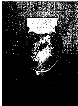
North Oakland Regional Sports Center-clogged toilet
