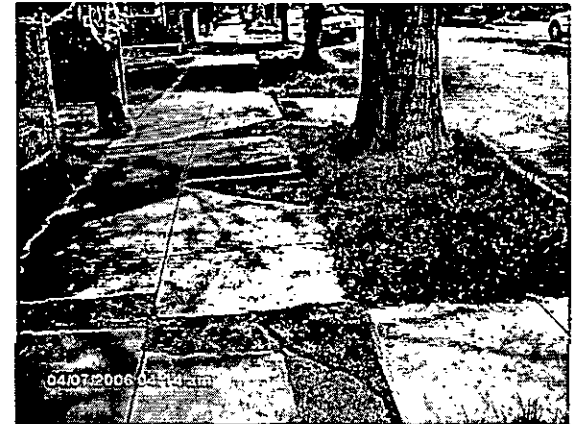
Tree Damage to Sidewalk
