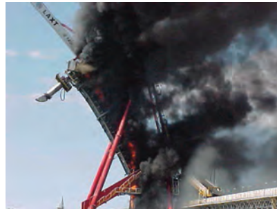
Figure 1: Shiploader during first fire.
