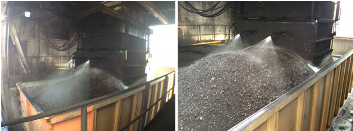
Machines contour and spray coal when loading on rail cars to prevent dust releases
