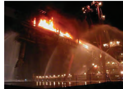
Figure 2: Shiploader during second fire
