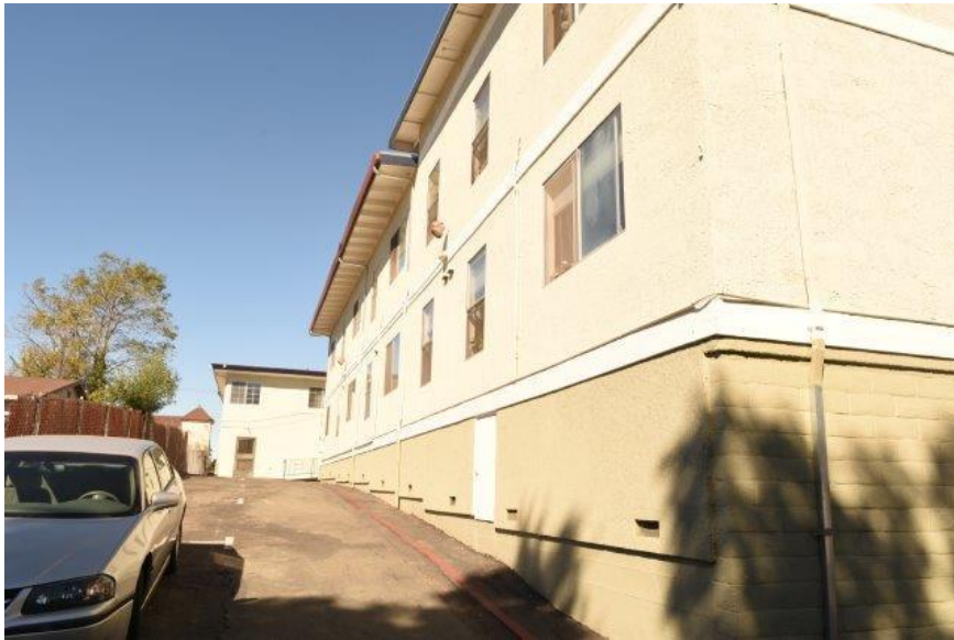
Figure 4 South Building's 2.5 story section
