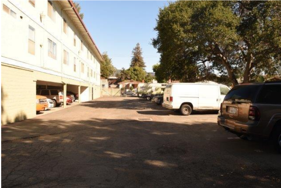
Figure 2 Parking lot and tucked under parking
