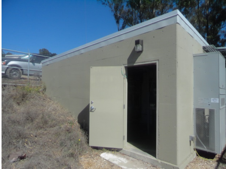
EBRCS shelter at Berkeley Labs
