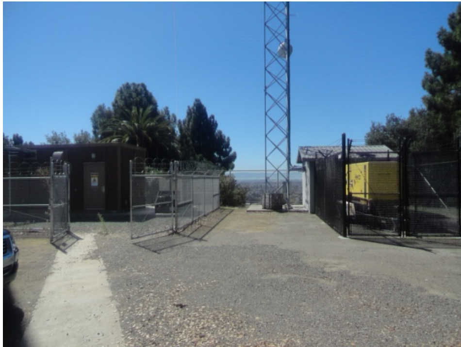
EBRCS shelter on left Oakland shelter on right at Seneca
