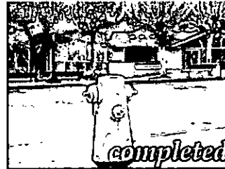
LAKESIDE PARK Fire Protection System
