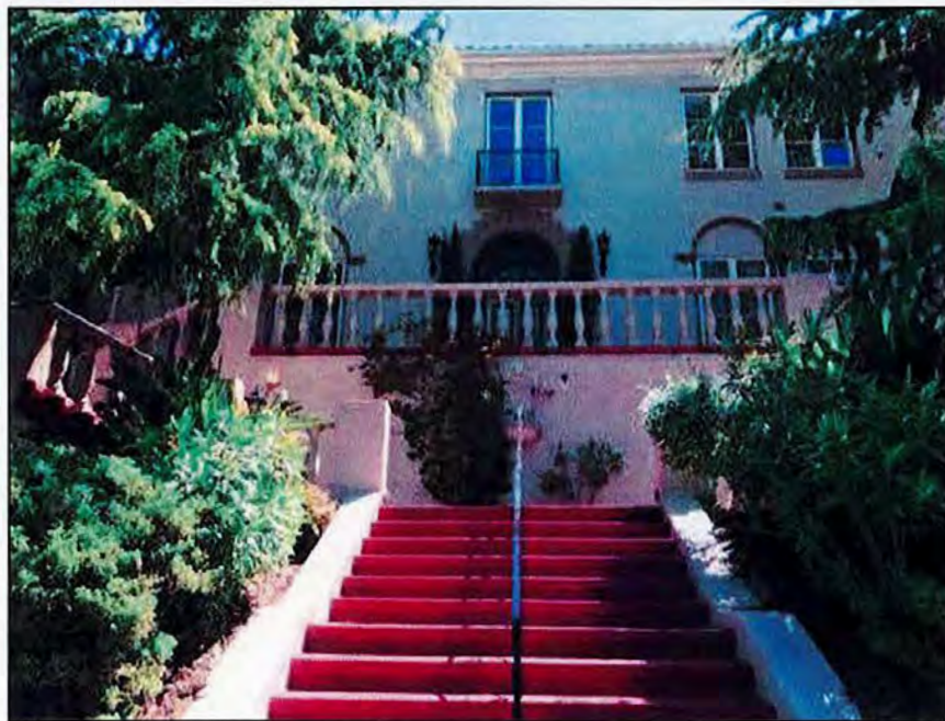
Figure 3. Detail of compound staircase, view east (SWCA, 2018).
