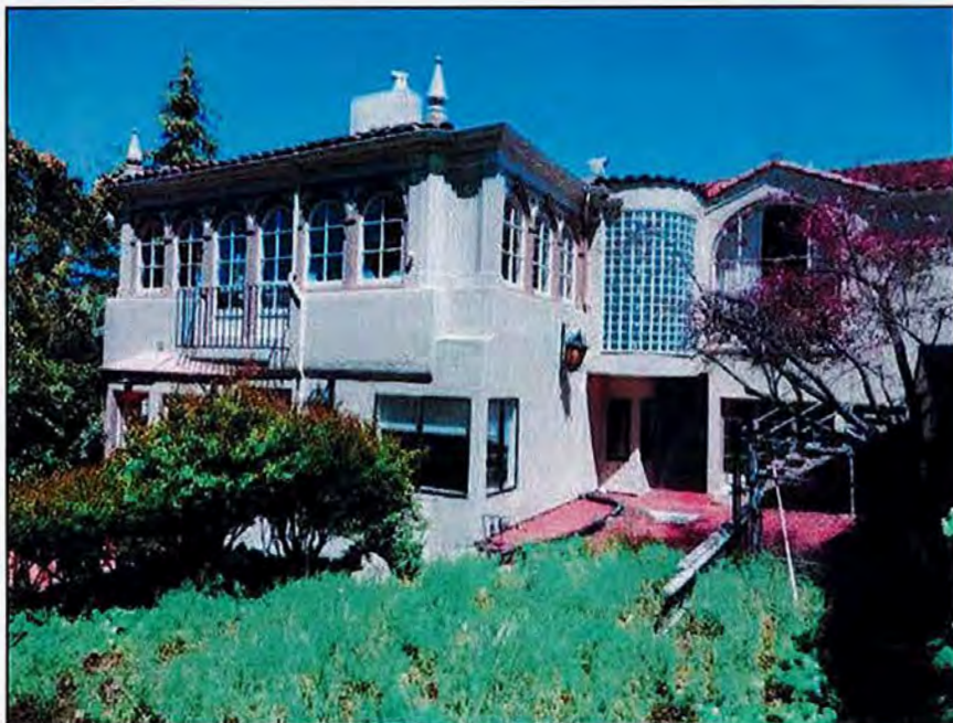
Figure 5. Overview of south façade, view north (SWCA, 2018).
