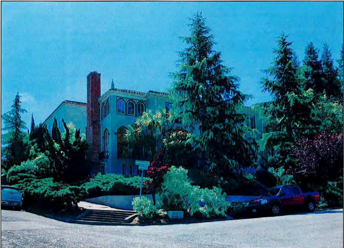
Figure 1. Overview of north and primary (west) façade at 664 Haddon Road, view east (SWCA, 2019).
