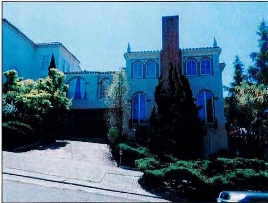
Figure 4. Overview of north façade, view south (SWCA, 2018).
