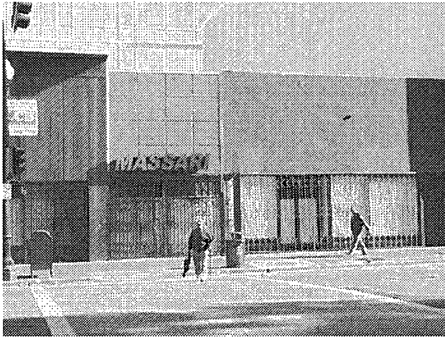
Broadway and Telegraph: unoccupied commercial buildings, deteriorated facades.
