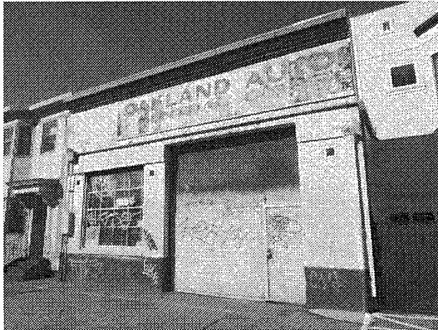
7th Street and Webster: abandoned, commercial building with vandalism, deteriorated signage and facade.
