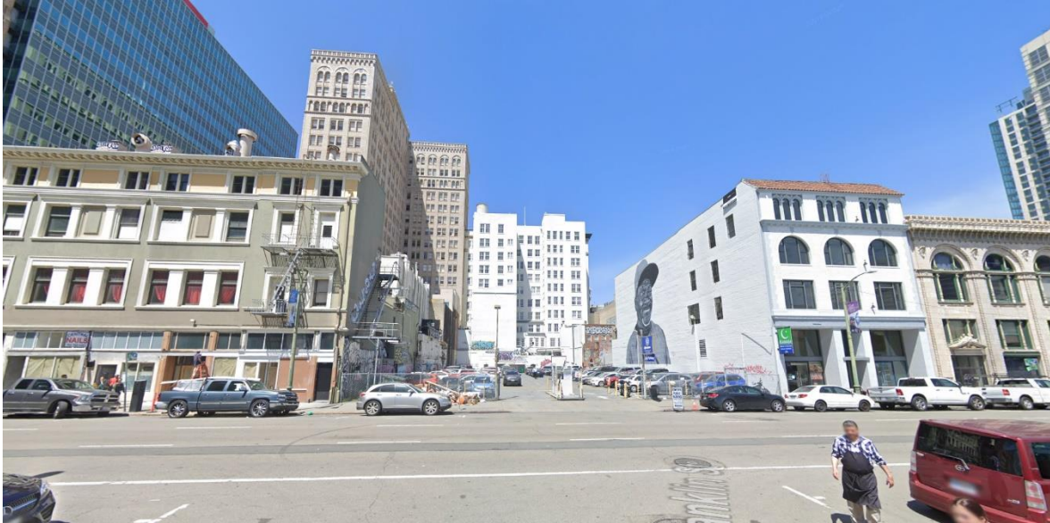
Photo of existing 1431 Franklin Street site.
