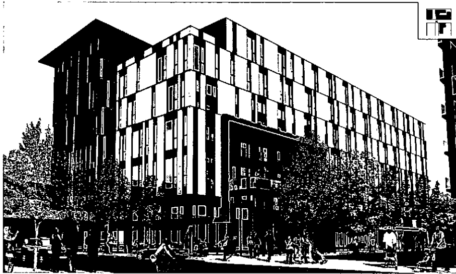
VIEW FROM INTERNAL STREET
