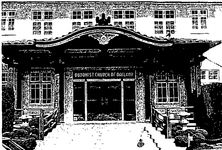
253-16 Entry Detail, 825 Jackson St., (S.W. corner 9th St.)
