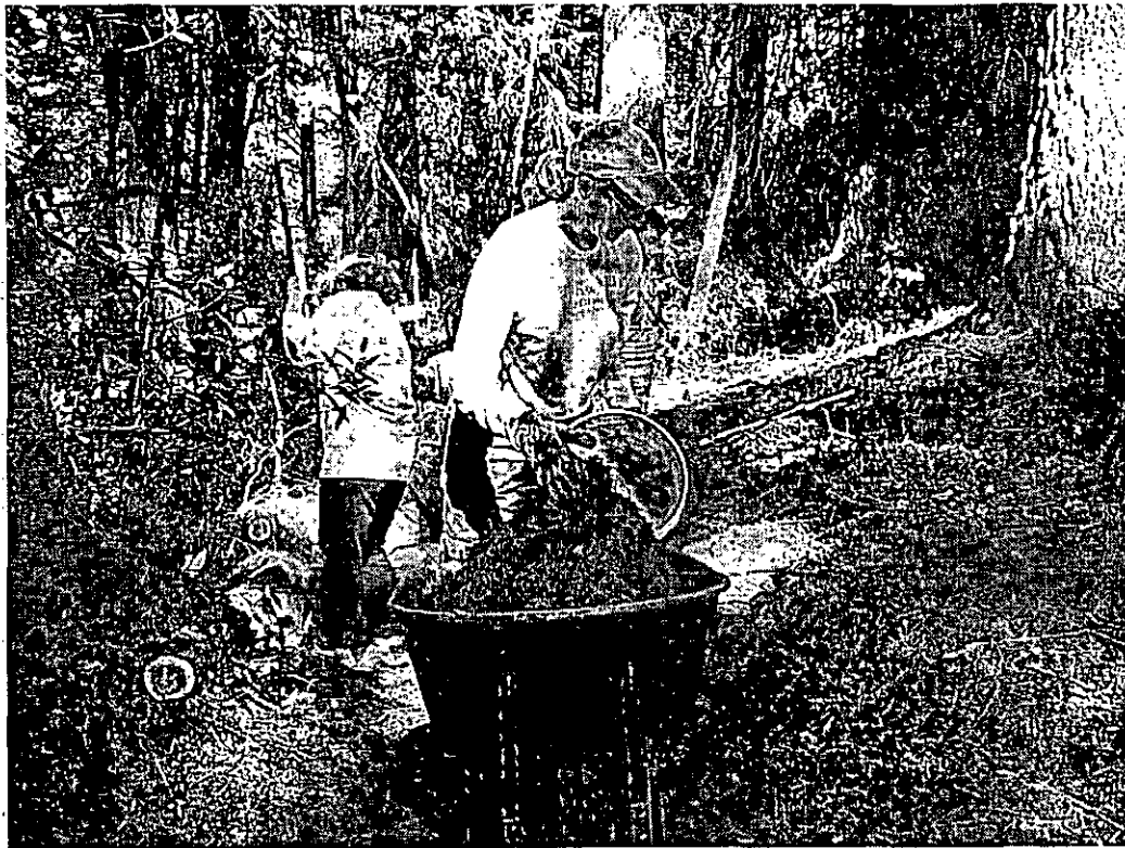
Removing duft on the new Big Trees reroute-- all by hand.
