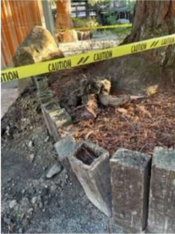
Existing Planter Box
