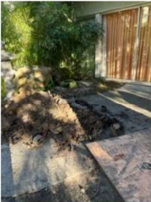
Recent Drain pipe repair.
