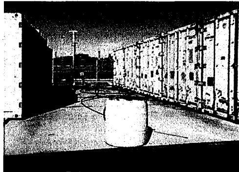
Elevated reefer cleaning pads
