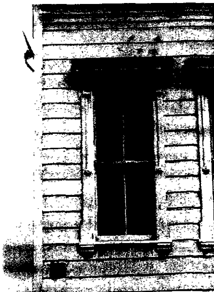
Photograph 17. Exterior window at 1970 San Pablo.
