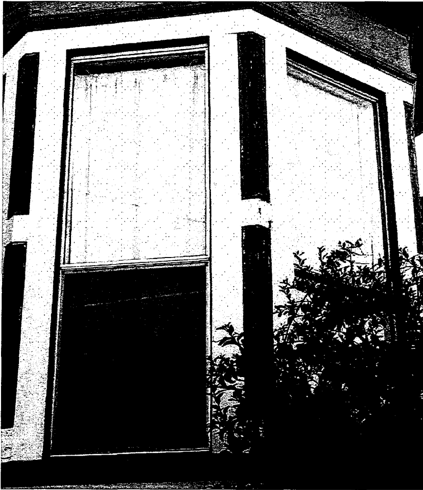
Image #5 One of the 12 aluminum windows to be replaced by original wooden windows Years 2023-2026 of the work plan
