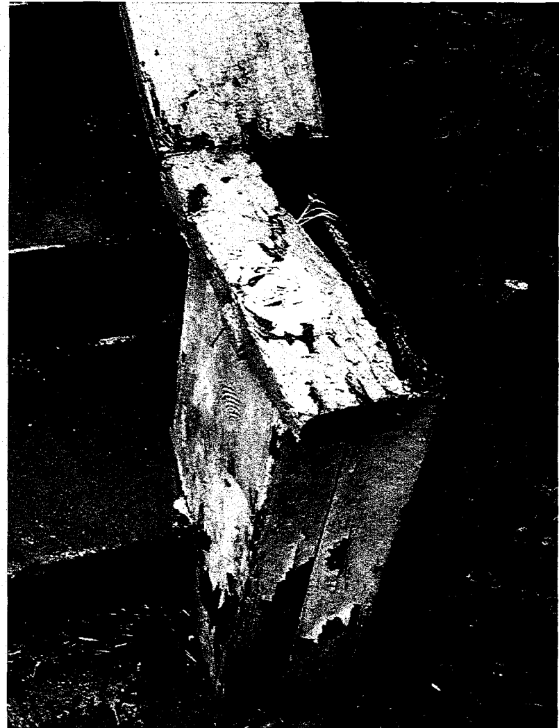
Image #2 Front stair wall to be rebuilt Years 2017-2019 of the work plan
