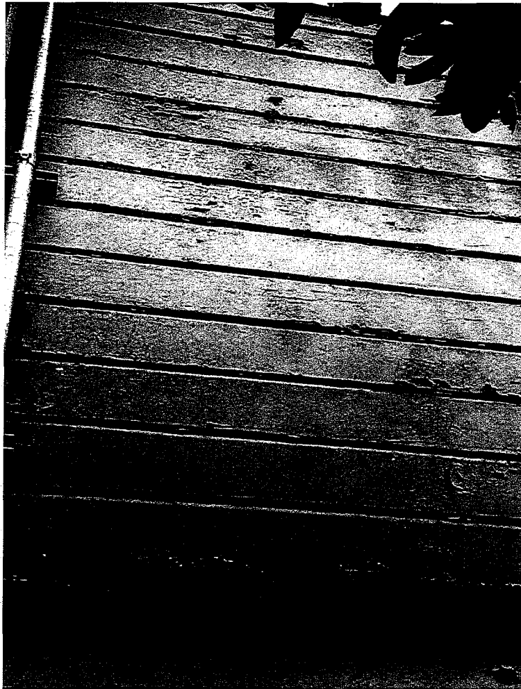
Image #3 An example of the exterior Siding to be scraped, sanded and painted (the whole house looks like this) Years 2017-2019 of the work plan
