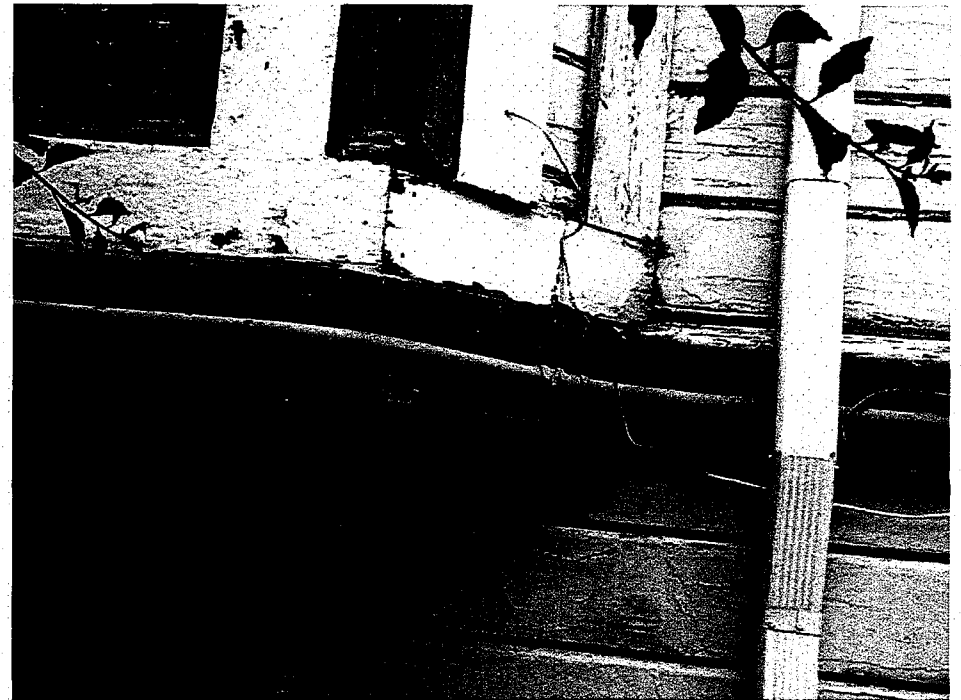
Image #4 Exterior dry rot, refastening and replacement of detailing (the whole house looks like this) Years 2017-2019 of the work plan
