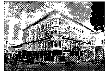
Built in the early 1870s, Eureka's Vance Hotel was wired for electricity by 1885. Restored and seismically stabilized, it houses retail, office, and commercial spaces.
