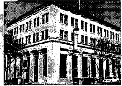
The Bank of Italy Building, Merced project involved removal of a non-historic facade, and rehabilitation of the 1928 bank building
