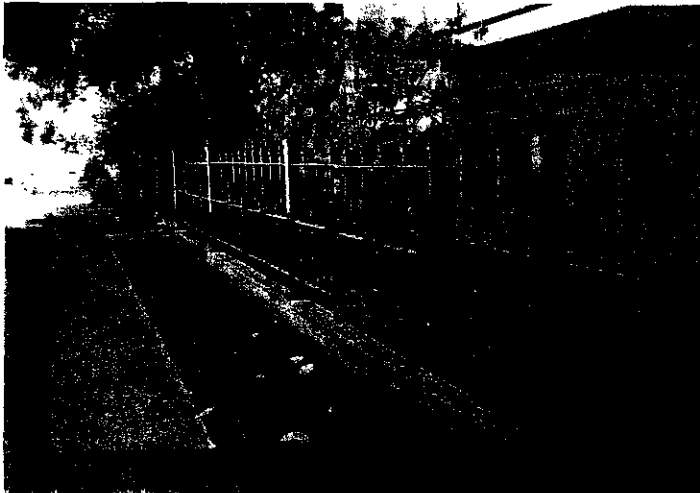
11.12 Consider a solid base up to about one foot high for wood or metal picket fences.
