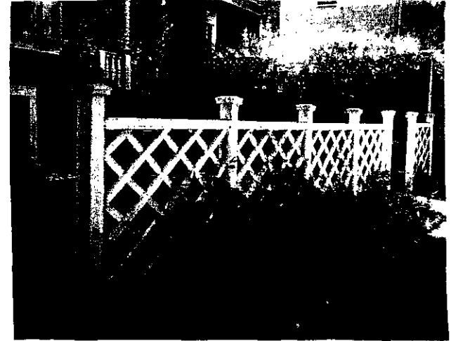
11.6 Set fences/walls out of the public right-of-way and at least 18" back from the sidewalk. Provide landscaping along the base of the fence/wall.
