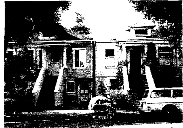
Fig. 8-5. The raised entry porches in this neighborhood create a strong transition between public and private spaces. In addition, all entry units are prominently located relative to the street.
