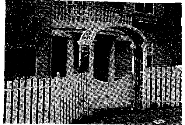
11.2 Use fence/wall designs that complement and are consistent with the architecture of the building.
