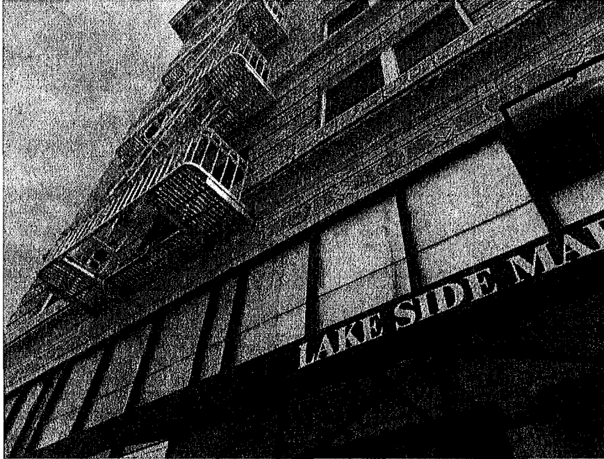
Figure 11. Photo showing brick and terracotta details.
