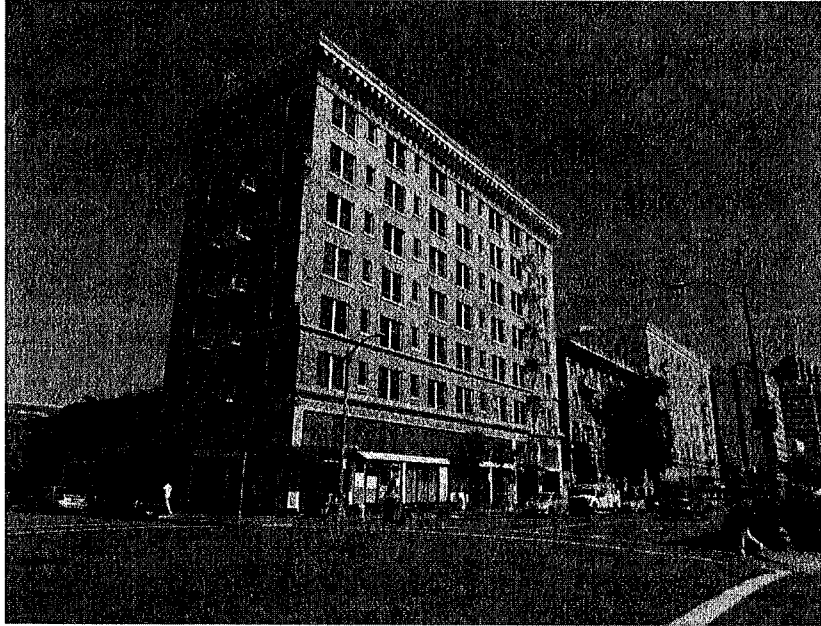
Figure 4. Photo showing the east and south elevations, facing north/northwest.
