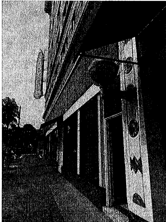
Figure 6. Photo showing the modified storefronts, clerestory, blade sign, and art deco style lights.
