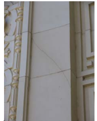
MINOR CRACK PATCH AND COAT
