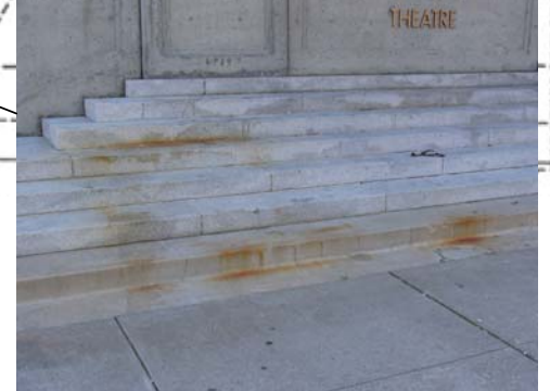
CORROSION STAINS AT GRANITE STAIRS
