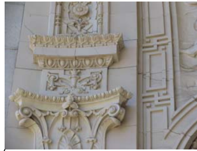
CRACK PATCH AND COAT
