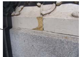
MINOR SPALL PATCH AND COAT
