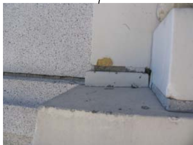
MINOR SPALL PATCH AND COAT
