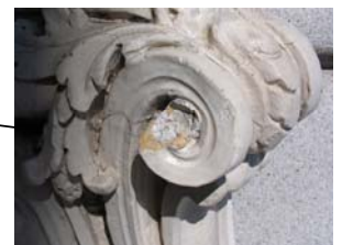
MINOR SPALL PATCH AND COAT
