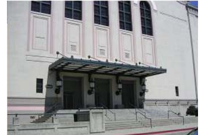
Existing east entry to be reused as library main entry
