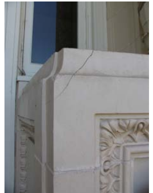
MINOR CRACK PATCH AND COAT
