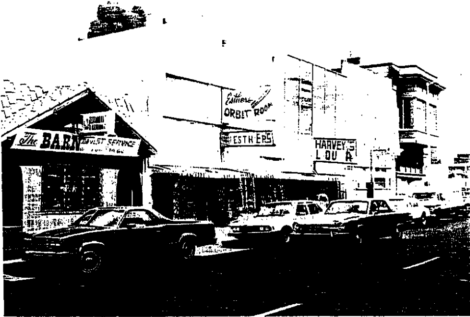
Photo No: 501-26 Date: 09/24/87 Location: 7TH STREET ASI VIEW EAST ON 7TH FROM 1726 7TH
