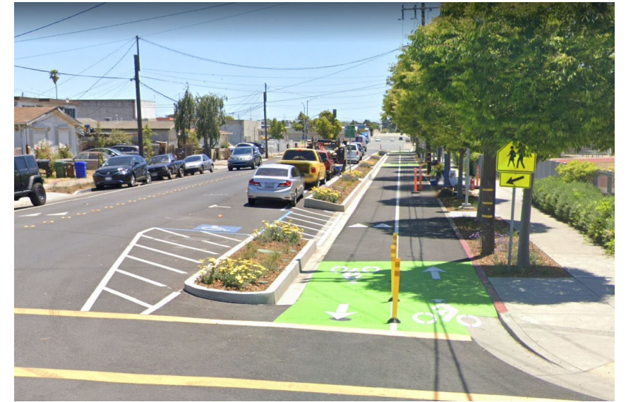
Example Facility – Marina Way, Richmond, CA
