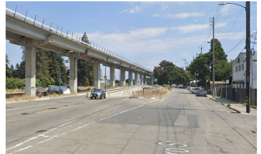
San Leandro Street tunnel at 105 th Ave
