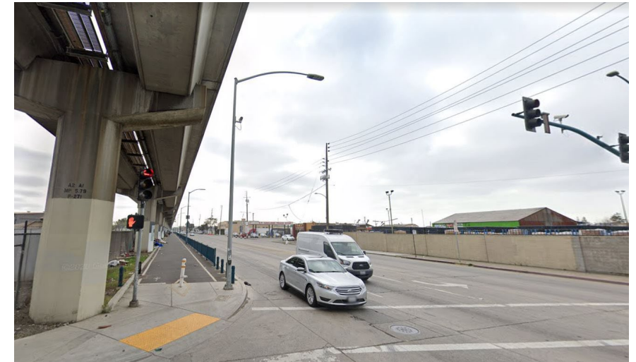
Example Facility – San Leandro St, Oakland, CA
